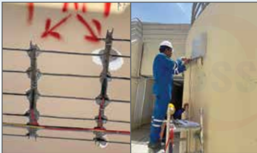
Installation of Anode System into slots cut into the concrete Surface
