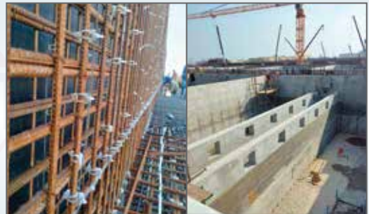
Installation of anode system on to rebar cage using non-metallic clip
